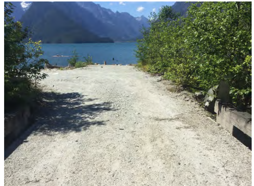
Left Approach Facing Away From Bridge
