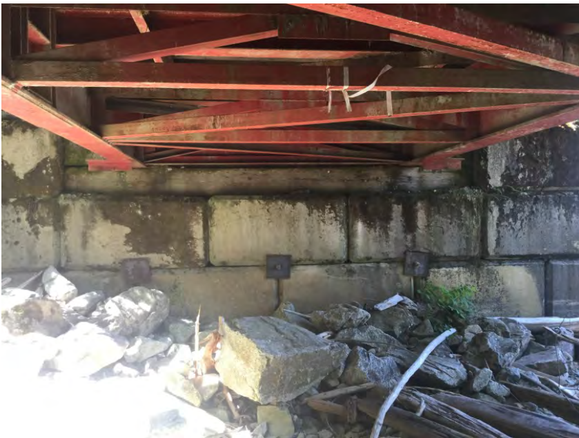
Left Bank Abutment
