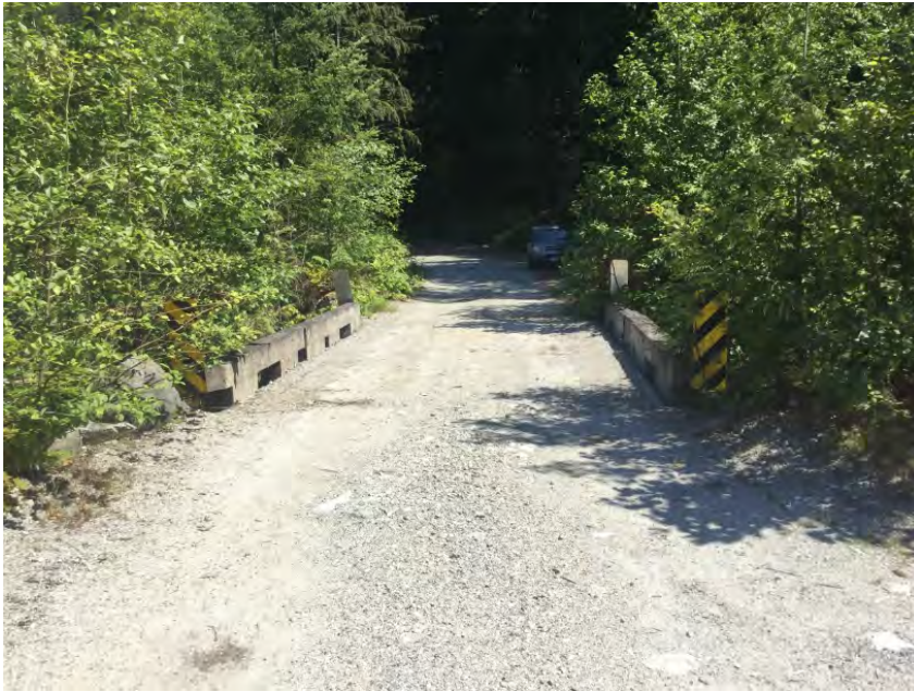
Left Approach Facing Bridge
