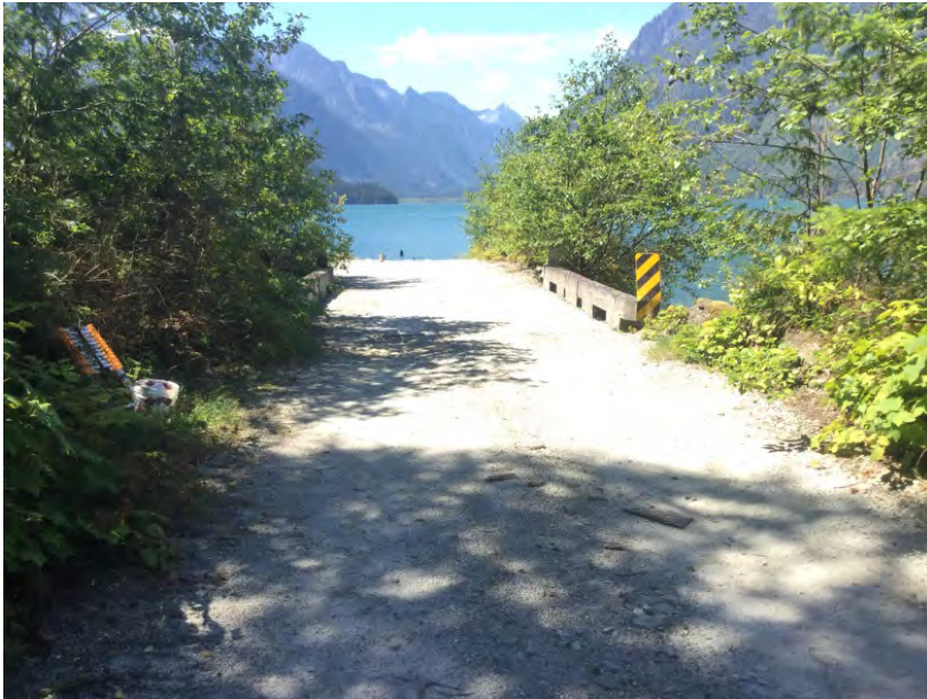
Right Approach Facing Bridge
