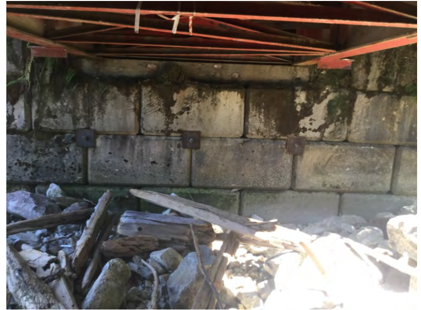
Right Bank Abutment
